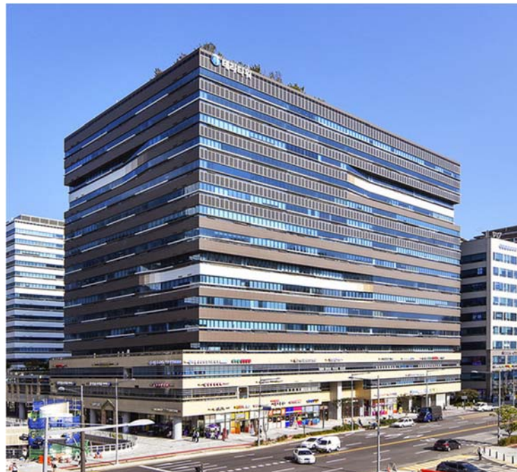
External view of building in which our Korean subsidiary is located
