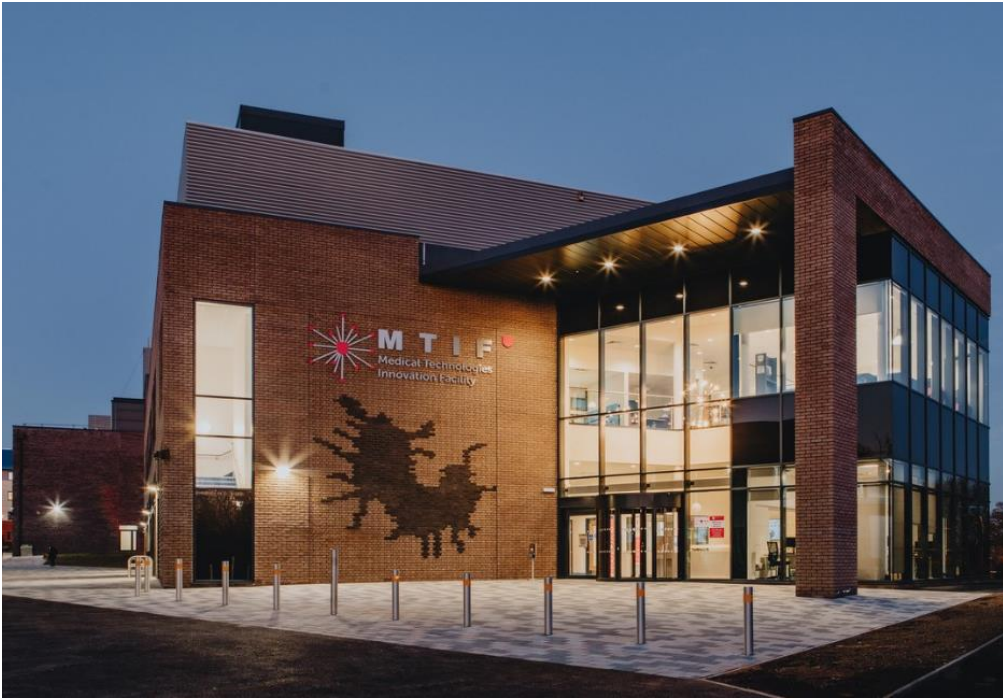
Medical Technologies Innovation Facility (MTIF)
