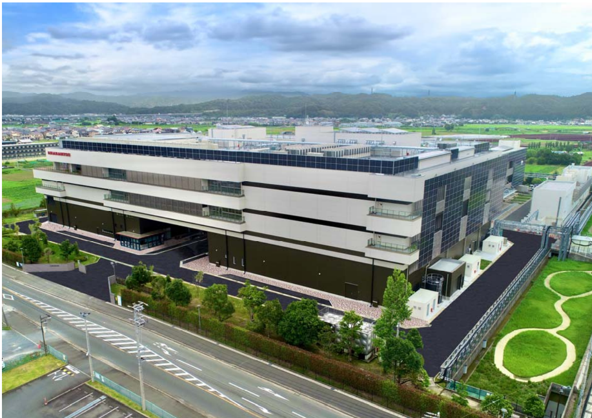
External View of Building No. 11 at our Toyooka factory
