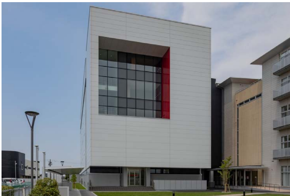
External View of Building No. 5 at our Joko factory
